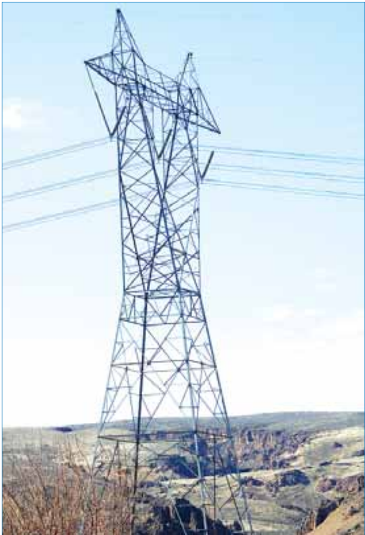
Towers on the Gateway West line will also be 500kV constructions much like these 150- to 180-foot towers on the PacifiCorp line that traverses Owyhee County, Idaho Power confirmed.
